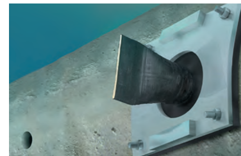
Retrofitted 4" square-flanged Tideflex® Diffusers to OD of RCP outfall with fixed-diameter ports
