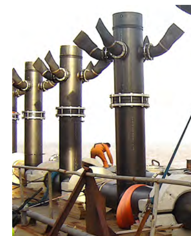
Tideflex® Diffusers discharge at an inclined angle to maximize dilution for dense jet brine outfalls from desalination plants
